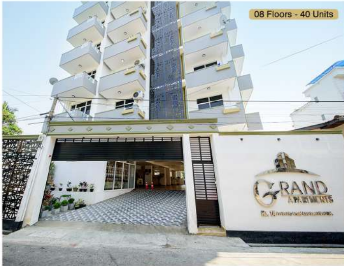
GRAND APARTMENTS No.14, Sri Wimalasiri Road, Dehiwala
